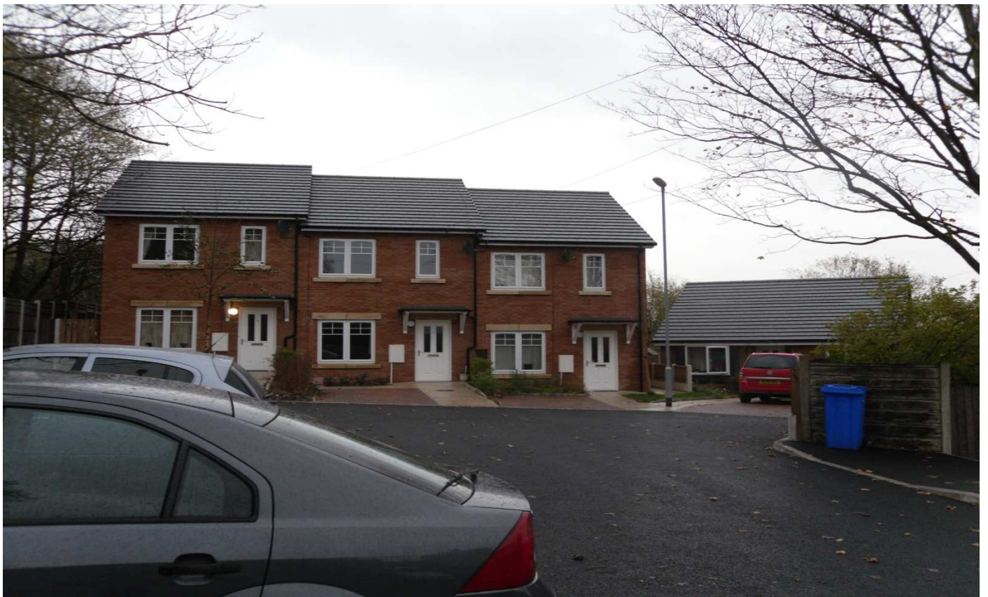
Taggwood / Hillside Road, Ramsbottom
